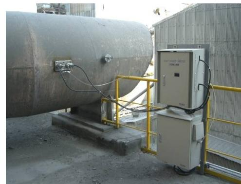
Detector head installed at duct open end.
