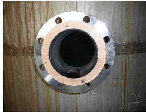
A hole making to the duct, and welding of probe attachment flange JIS 10K 100A (standard size)
