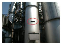
The installation of the DDM-fC is simple and costs you less. To install the detector you need just one hall on a stack and minimal work space.
