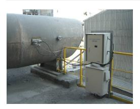
Detector head installed at duct open end.
