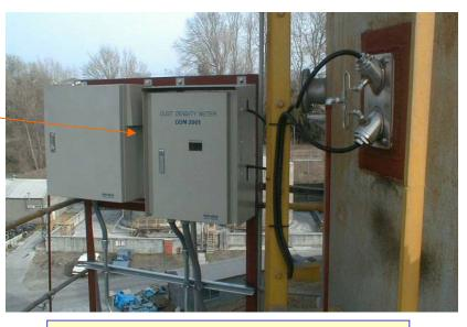
AQC(Air Quenching Cooler) EP outlet stack
